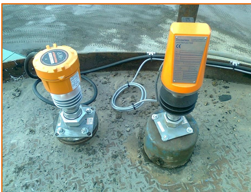
Pictured: High-temperature Hycontrol TDR probe and RF Admittance switch in a bitumen application
