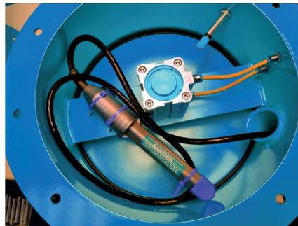
Figure 5: Shows level probe sensor underside of PRV secured by 3 cable ties and with tip protector
